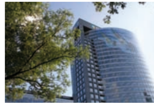
In the ABN-Amro Bank in Amsterdam, an EY3600 system handles extensive control tasks. Smooth operation is guaranteed thanks to an in-house technical maintenance team coupled with Sauter's 24-hour stand-by service.
