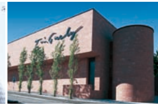
The Tinguely Museum in Basle is dedicated to renowned iron sculptor Jean Tinguely (1925 - 1991) and is controlled by a Sauter EY2400 system that has operated virtually without faults for a good ten years – thanks to regular maintenance by Sauter.
