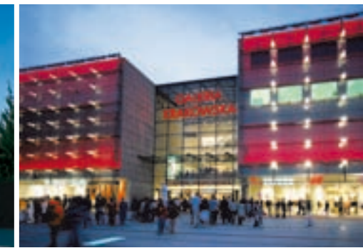
Galeria Krakowska is the largest shopping centre in Cracow, Poland; Sauter Slovakia installed the building automation system, so the same firm was entrusted with the maintenance, which includes one minor and one major service each year.
